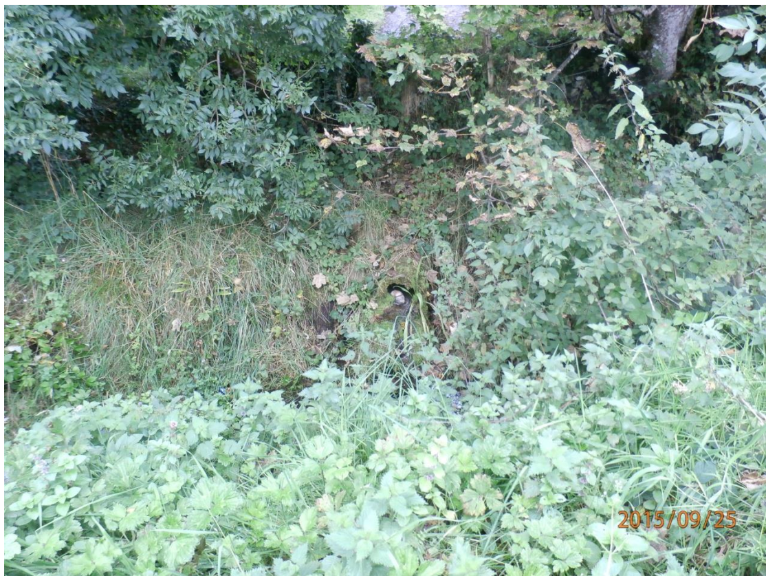
Pipe crossing N15 and discharging into drain from Spring Cotton Wool sample collected to establish groundwater flow from Swallow Hole No 2 Collecting: 25/09/2015
