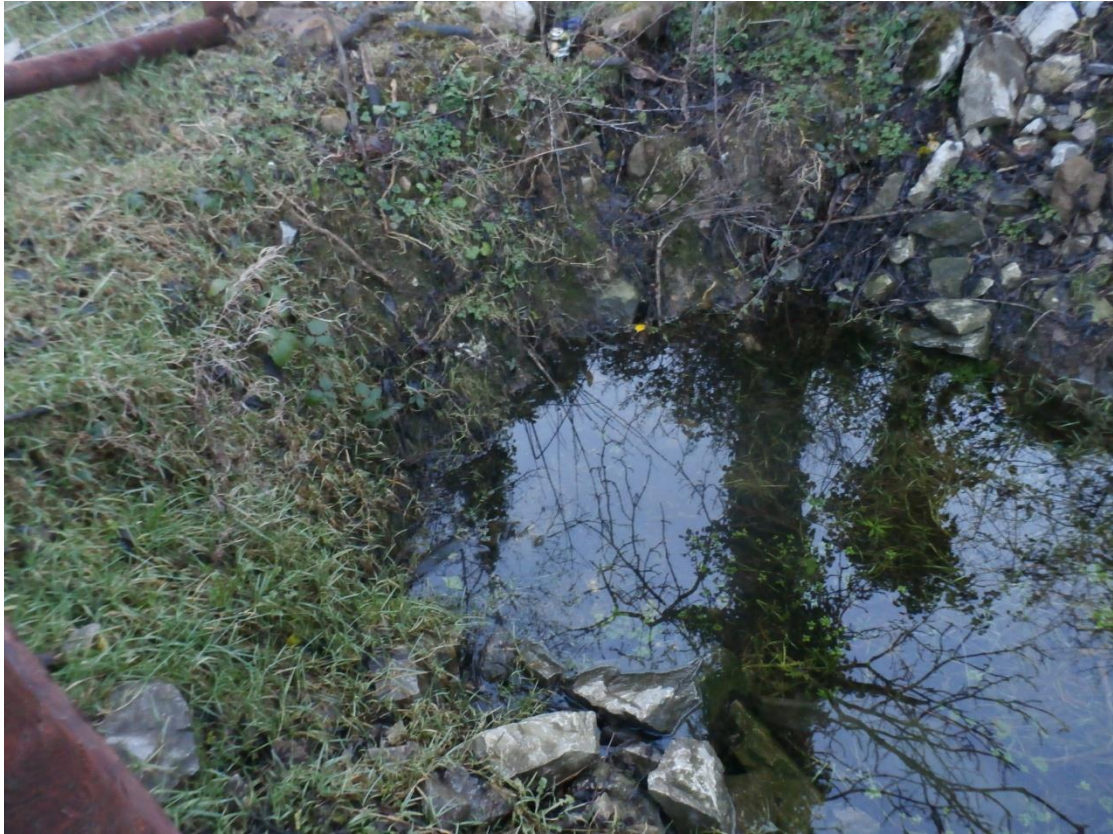
Swallow Hole adjacent to Swallow Hole No 1- Point ID 81 invert level 83.481mOD Swallow Hole working January 2015
