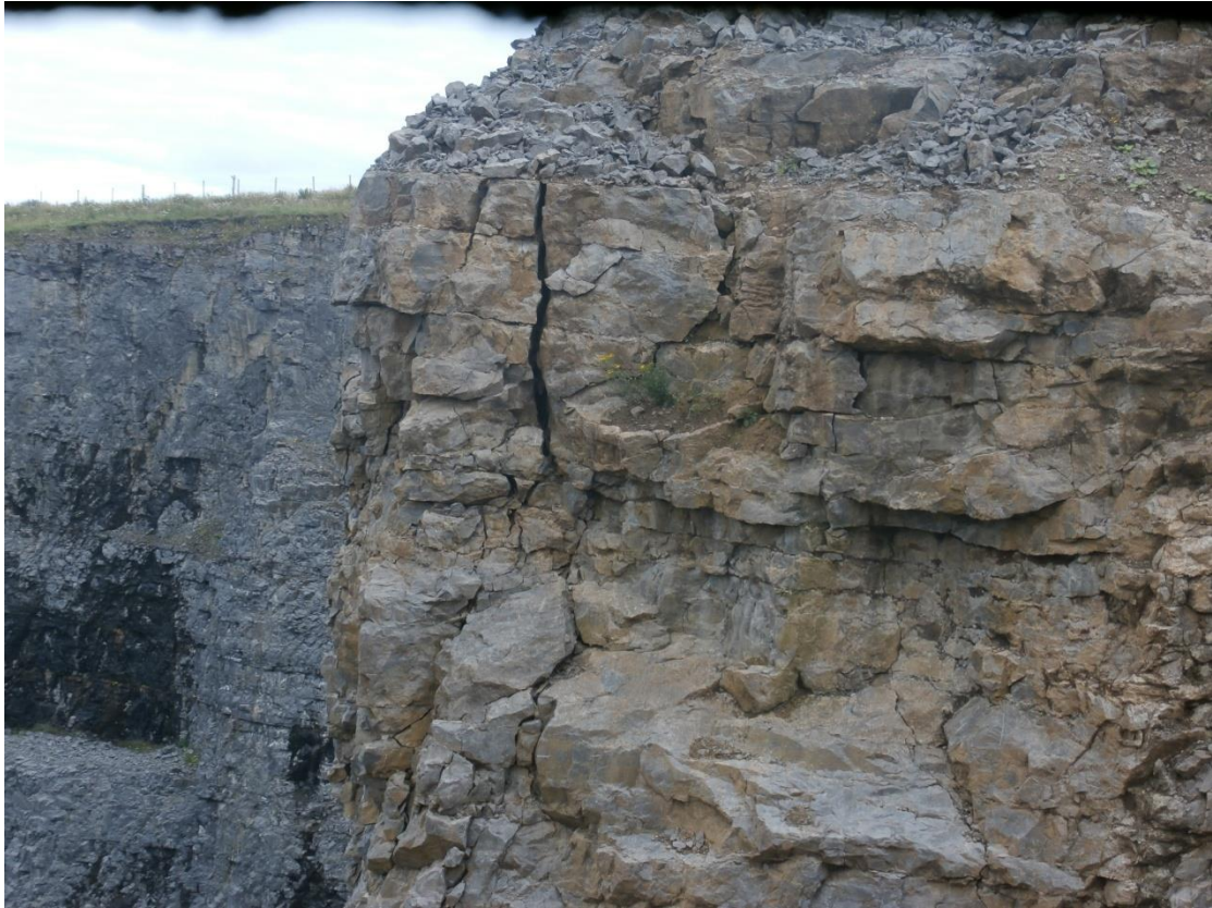
Photograph of west face of north quarry with cracks through rock face 07/08/2015
