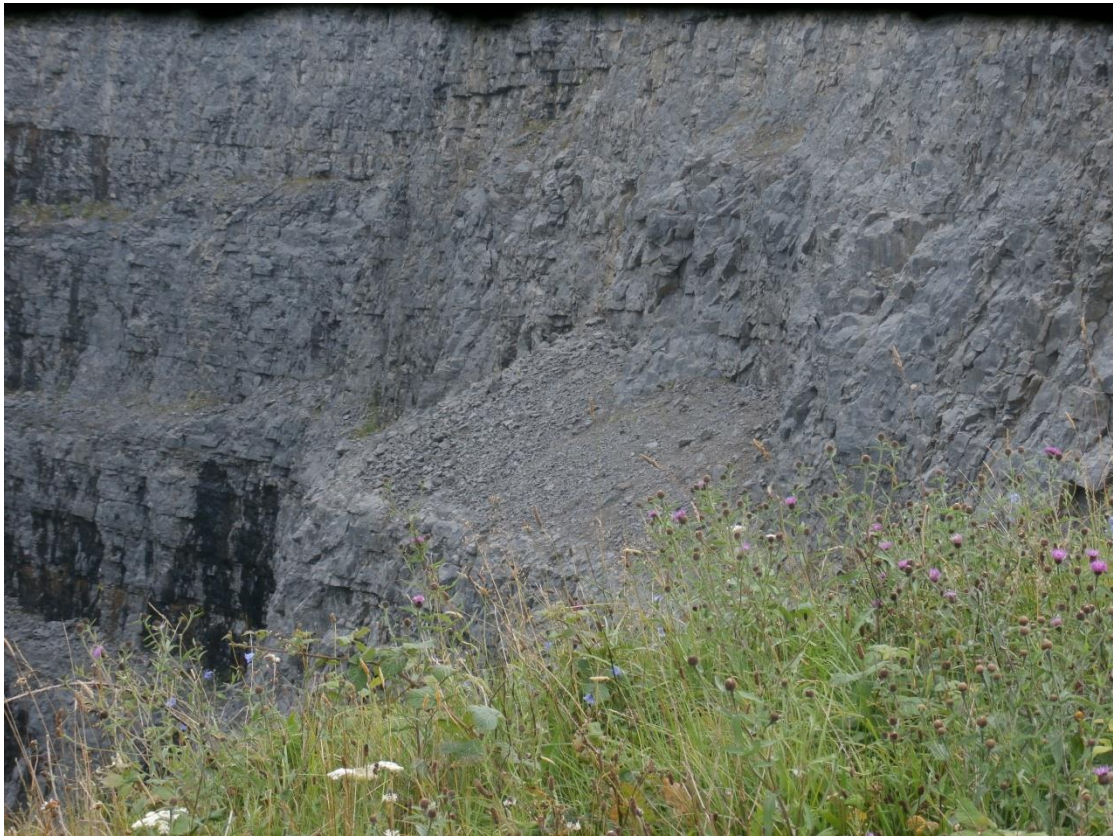
West face of north quarry 07/08/2015
