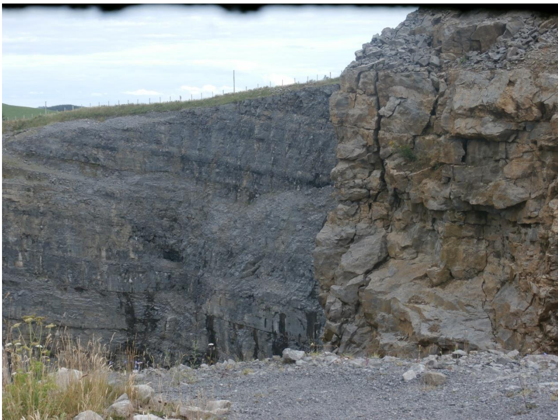
West face of north quarry with cracks through rock face 07/08/2015
