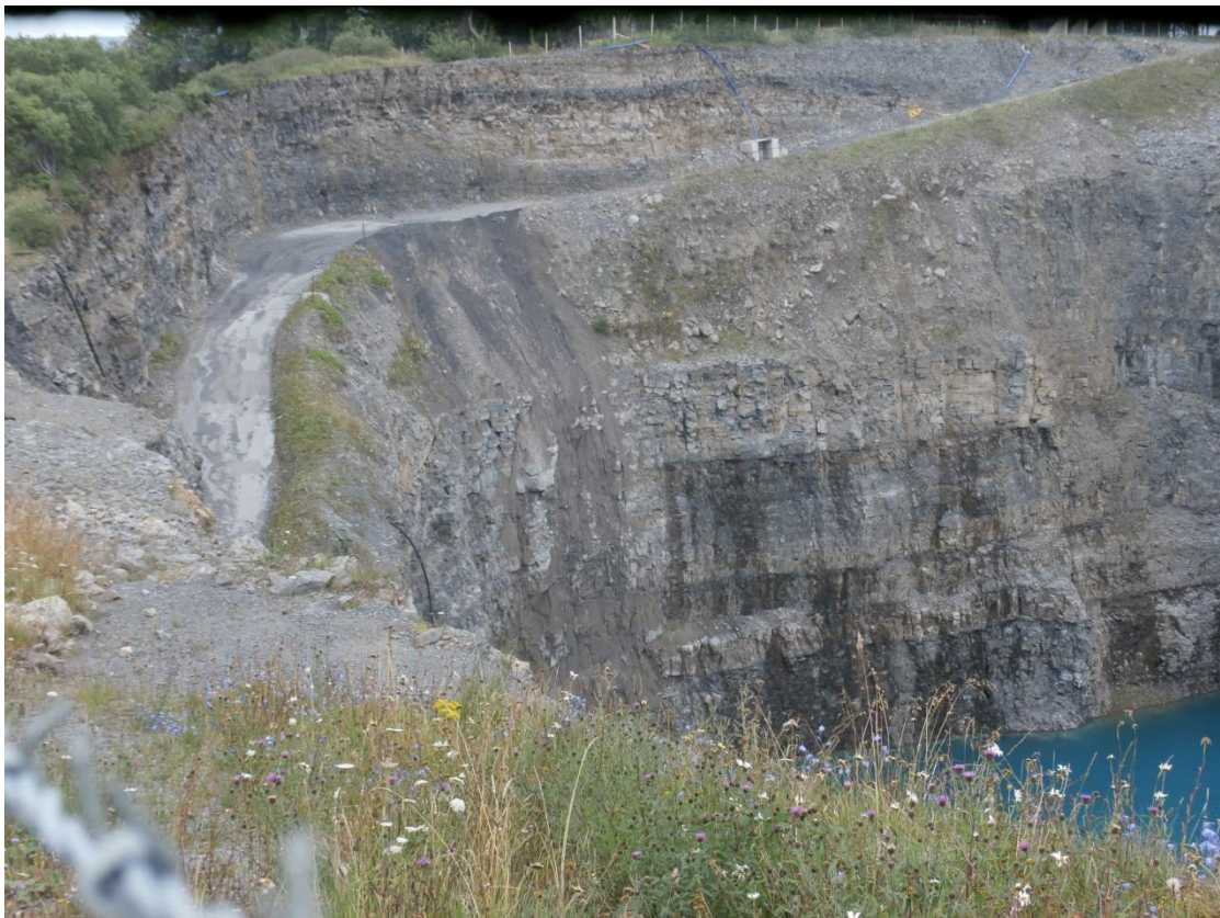
Access road into north quarry with deposition from unauthorised dumping on cliff face 07/08/2015
