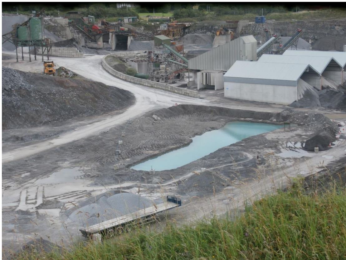
South Quarry – additional pond recently excavated in floor of quarry 07/08/2015
