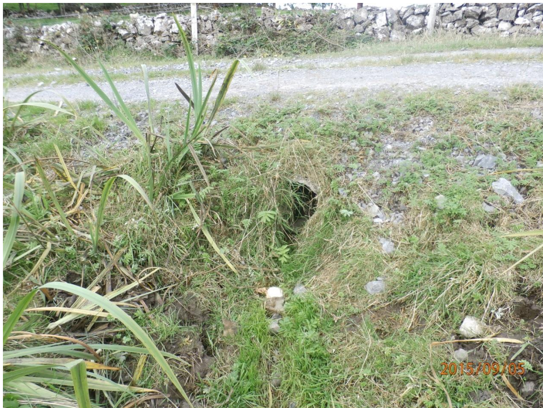
Underpass Cotton installation on 05/09/2015
