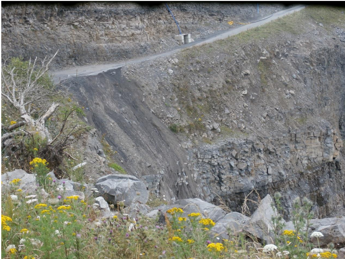
Access road into north quarry with deposition from dumping 07/08/2015
