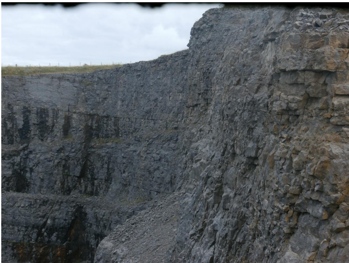
West face of north quarry 07/08/2015
