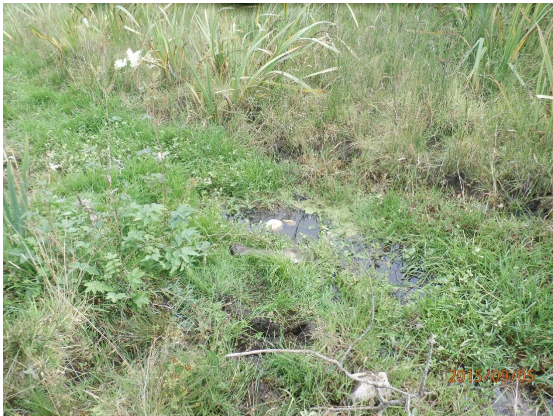
Drain in field on west side of access road Cotton installation on 05/09/2015
