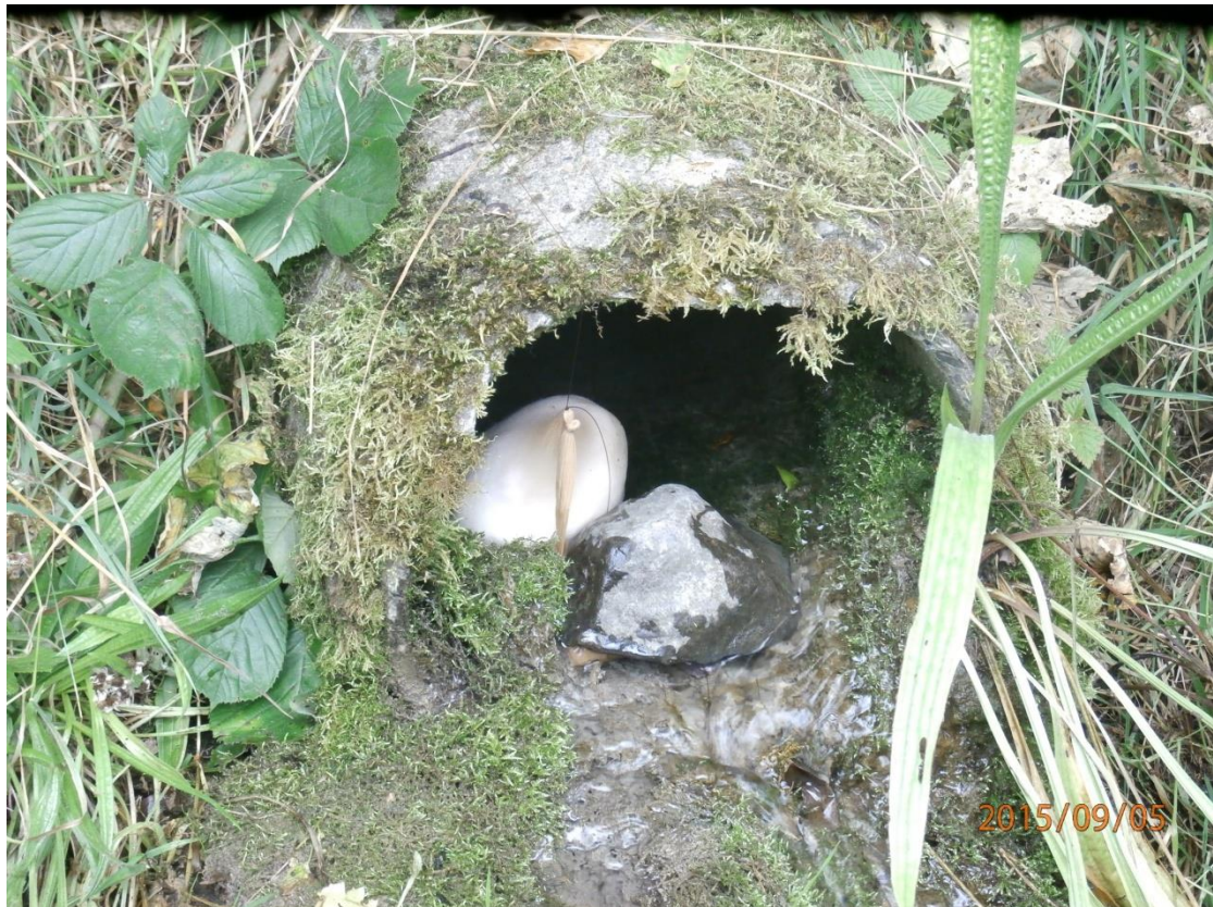
Pipe crossing N15 and discharging into drain from Spring Cotton placed to check clear Installing: 05/09/2015
